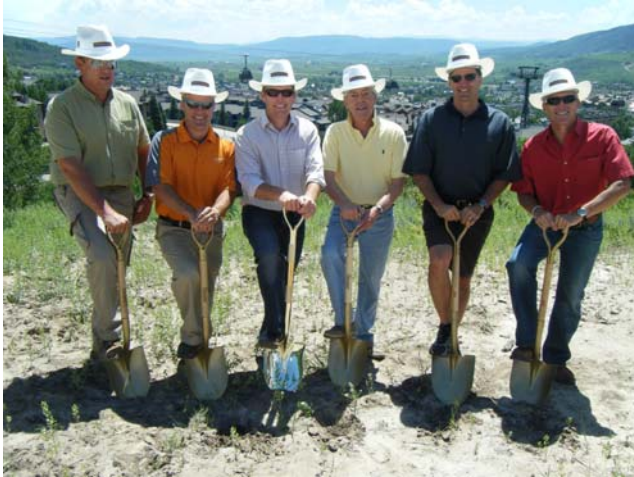
Edgemont Groundbreaking – From left are Mark Murrell (S&P Destination Properties, Sales Director for Edgemont), Eric Entlich (The Atira Group, Construction Manager for Edgemont), Garrett Simon (The Atira Group, VP of Development), Joe Brennan (Property Owner), Loui Antonucci (Steamboat Springs City Council President), CJ Berger (Summit Investment Management). — Courtesy Photo
