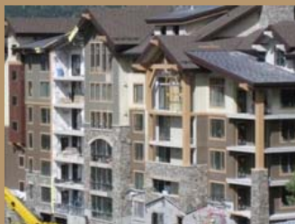
The Scaffolding Comes Down! 8/26/09
